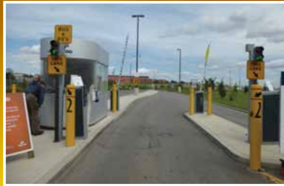
An entry lane into the 1,800-vehicle lot. The readers are visible just past the bollard marked "2," and the gates are at the end of the kiosk.
