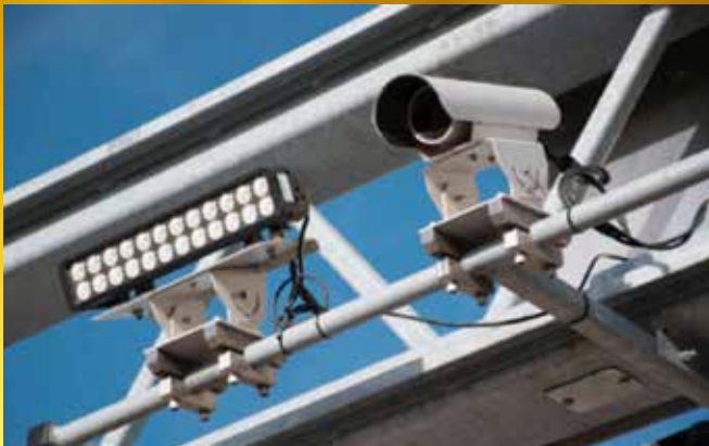
A close-up of the camera and light. Because Alberta license plates are non-reflective, LED lights are quite bright at 20,000 lumens.
