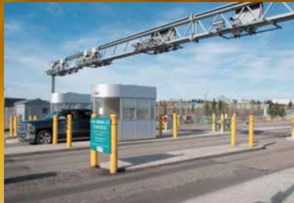
The new system in operation. The system went live just 10 days from installation of the gantry, wiring, cameras, lasers, and control cabinets.
