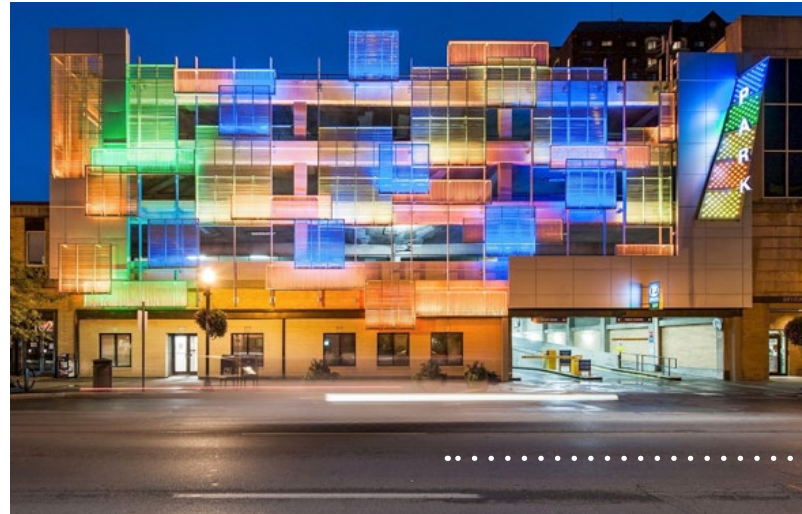
Stainless-steel façade panels and programmable LED lighting made the award-winning Helix Parking Structure a public art destination.
