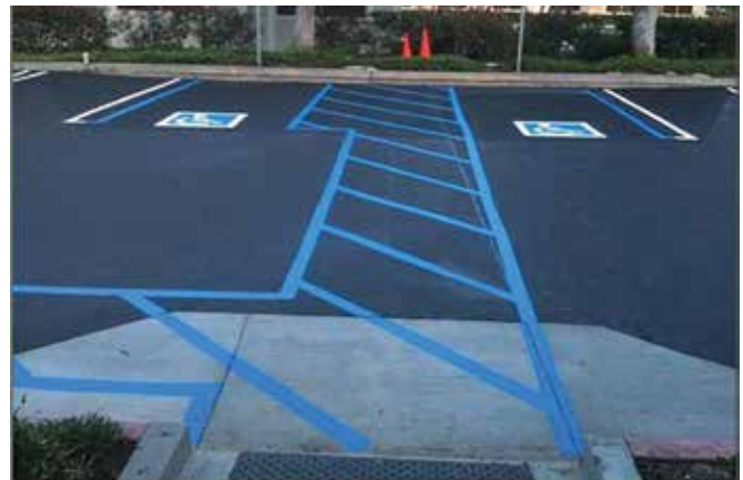
"502.3.2 Access Aisle Length. Access aisles shall extend the full length of the parking spaces they serve."
