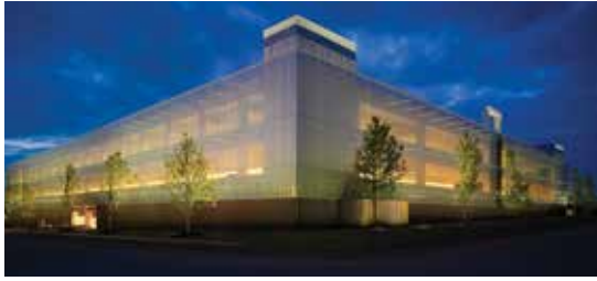
Car Park Two at Chesapeake, Oklahoma City, Okla.
