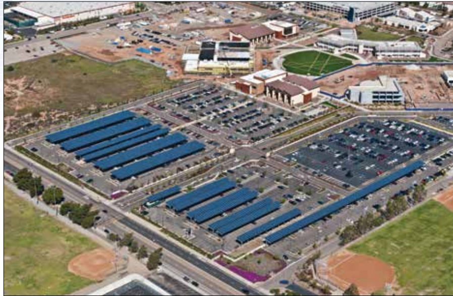
Solar installations on parking structures and over lots can save money and offer additional benefits to facility owners.
