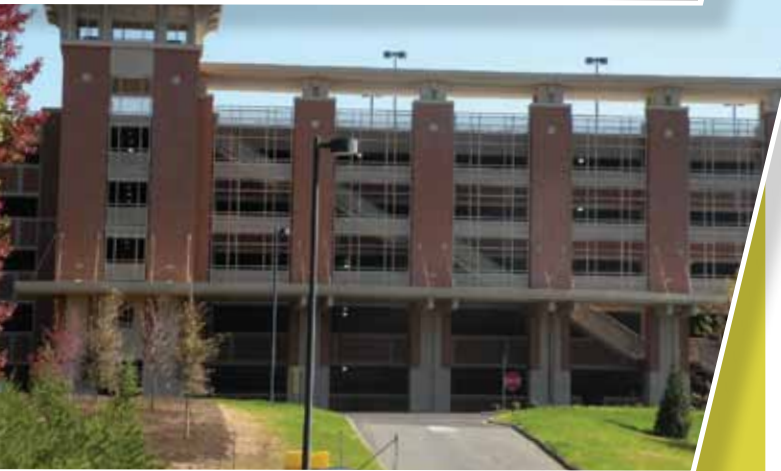
The UNC Charlotte Student Union Parking Deck was designed to be flexible and accommodate present and future campus development.
